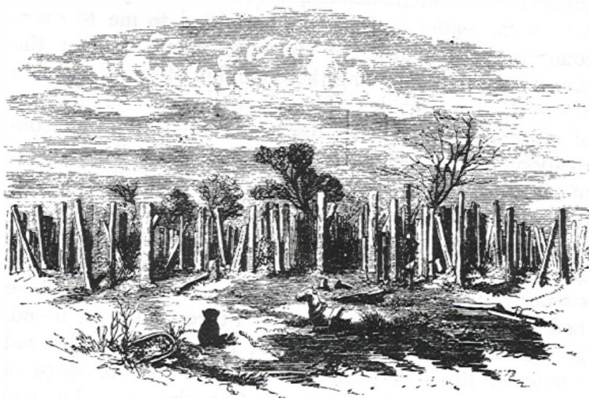
Fig. 6.2: Lohapāsāda, Anurādhapura, Sri Lanka: colonial-period view. The description of the Lohapāsāda in Chap. 27 of the Mahāvamsa , 'Consecration of the Lohapasada', is one of the most detailed descriptions of an ancient building in surviving records of South Asia. After James Emerson Tennent, Ceylon: An Account of the Island , London: Longman, Green, Longman, and Roberts, 1859.
